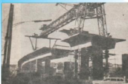
Seied Khandan (Tehran) bridge under Construction by using pre-stressed steel cables to join the prefabricated pieces (Date of construction: 1973)
